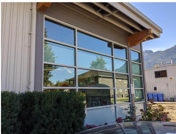
Windows at children's area (facing Municipal Hall to the north).
